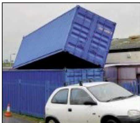
● A shipping container was dislodged by heavy winds at Shirehill (Photo: Ben Warbey)
